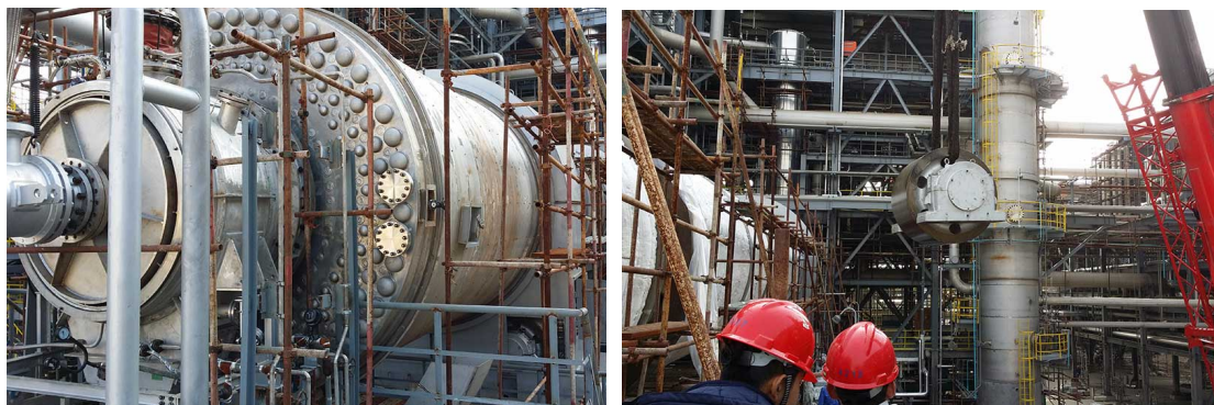
Environmental Protection Project Equipment Installation and Commission Site
