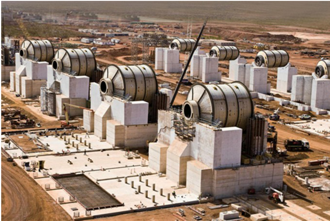
This is the installation site of \Phi 5 \times 8\text{m} autogenous mill and \Phi 4.9 \times 10.6\text{m} overflow ball mill produced for Sino Iron Ore in Australia
