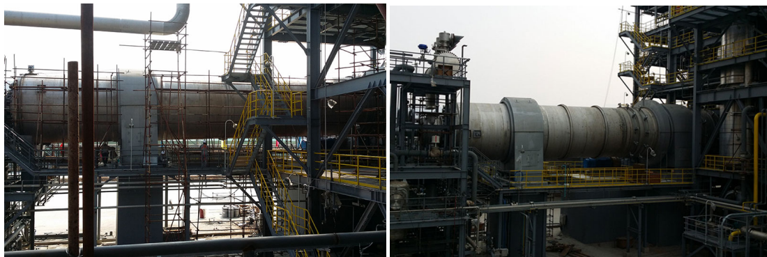
Installation and Commissioning Site of Rotary Dryer
