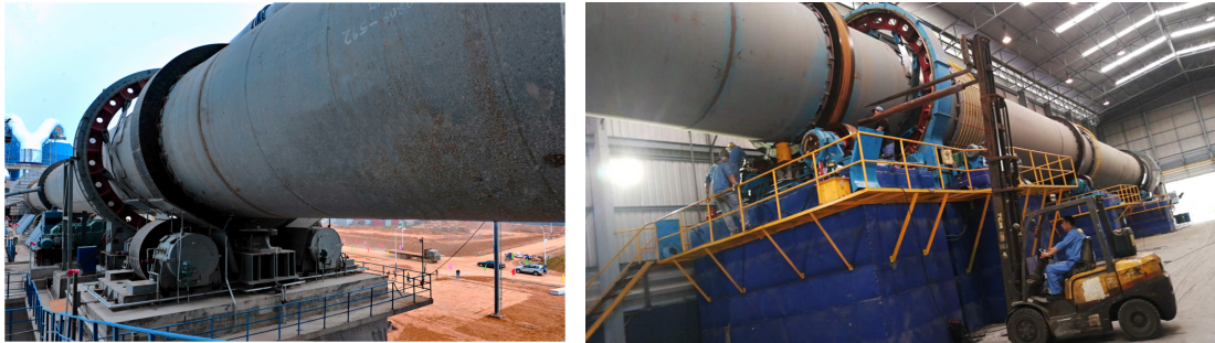
Installation Site of Rotary Kiln
