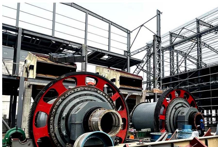
Φ3.8x5.0m Rod Mill Installation Site
