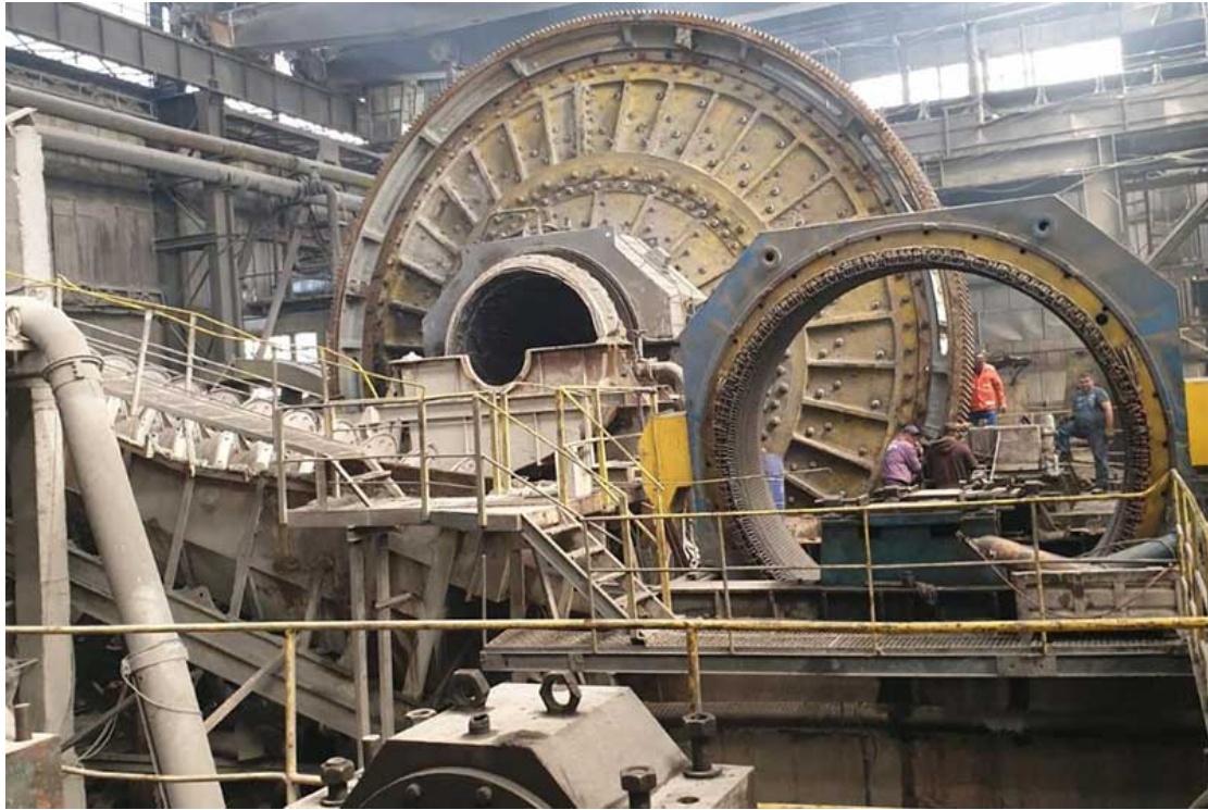
Commissioning Site of SAG Mill in Romania
