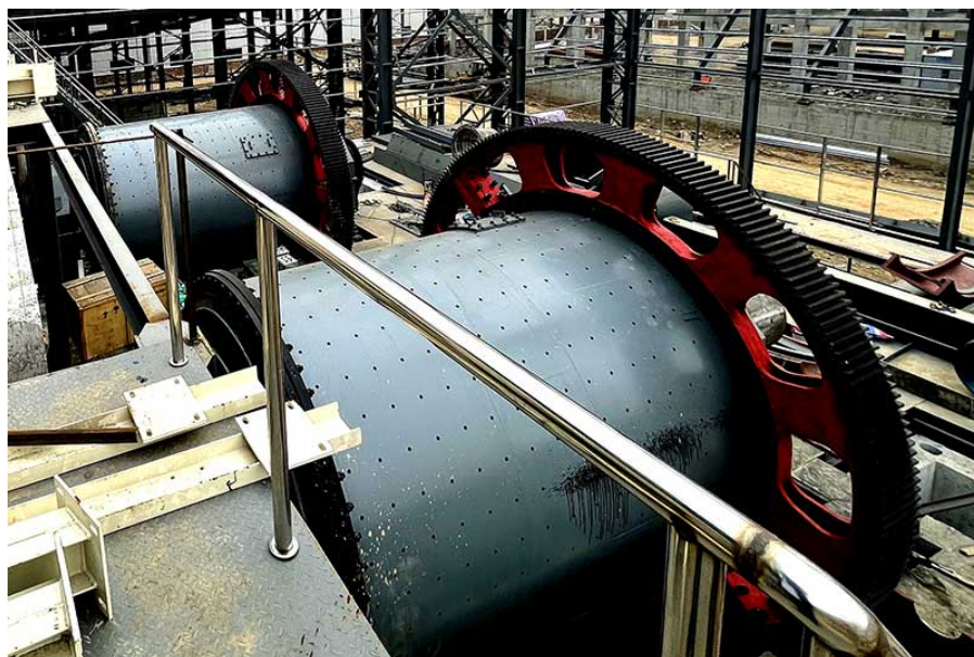
Φ3.8x5.0m Rod Mill Installation Site
