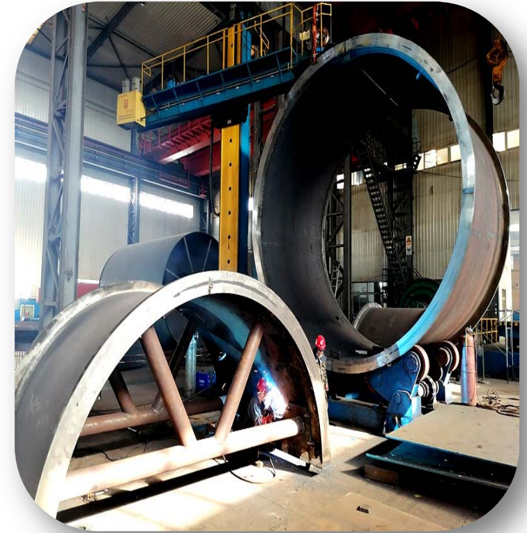
◆ Submerged Arc Welding
