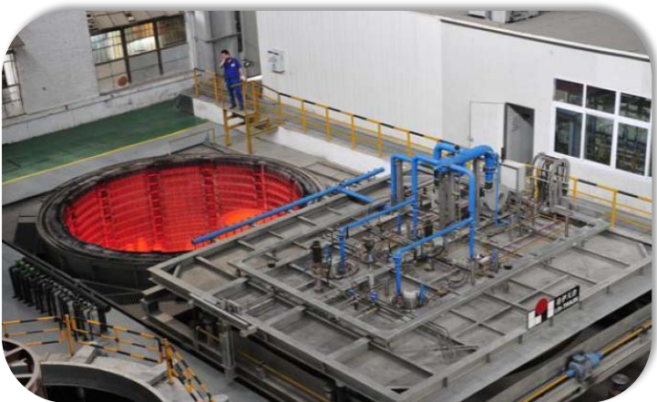
◆ \phi 5 \times 2.5 m Well Heattreatment Furnace
