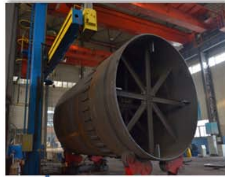
埋弧自动焊 (焊缝UT) Submerged-Arc Welding ( UT)
